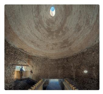
learn about the historical ice trade. New access elements were introduced, including an observation deck and staircase in Well 11, as well as a walkway spanning the void in Well 13. These elements, crafted from wood, deliberately contrast with the original materials.
