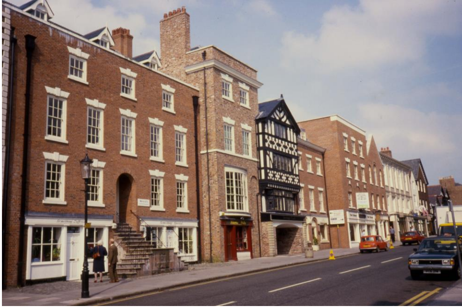
Lower Bridge Street after restoration.
