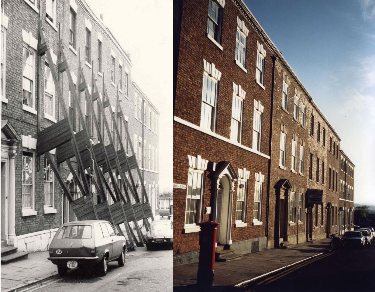
King's Buildings : Structural problems resolved
