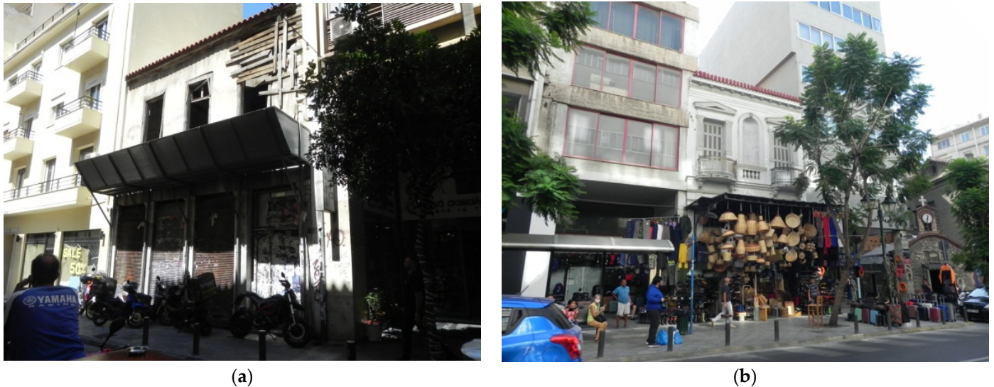
Figure 19. Photos of the area depicting the coexistence of different building types in the area of the Historical Commercial Triangle: (a) An abandoned two-story neoclassical building with significant damage next to a well preserved, typical Athenian's modernism building, Perikleous St. (b) A neoclassical two-story house with a shop on the ground floor next to a modern multi-story building with a gallery in the entrance, Athinas St.
