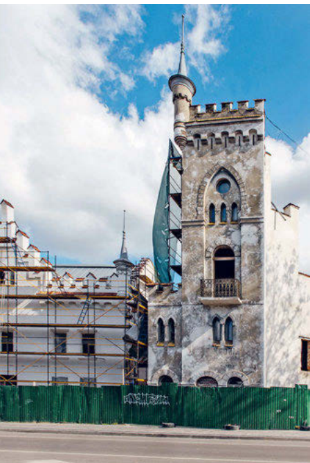
Fig. 5 Ongoing restoration and construction
