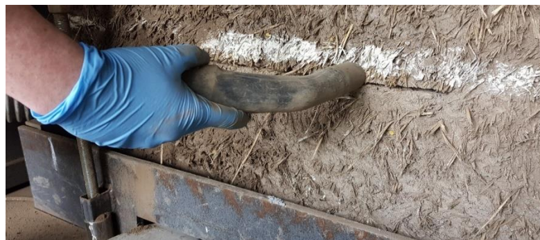
Figure 5. 52. Cleaning of the slot.
