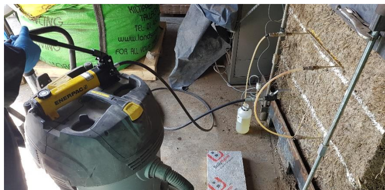
Figure 5. 62. Purging of the system with both flat jacks connected.
