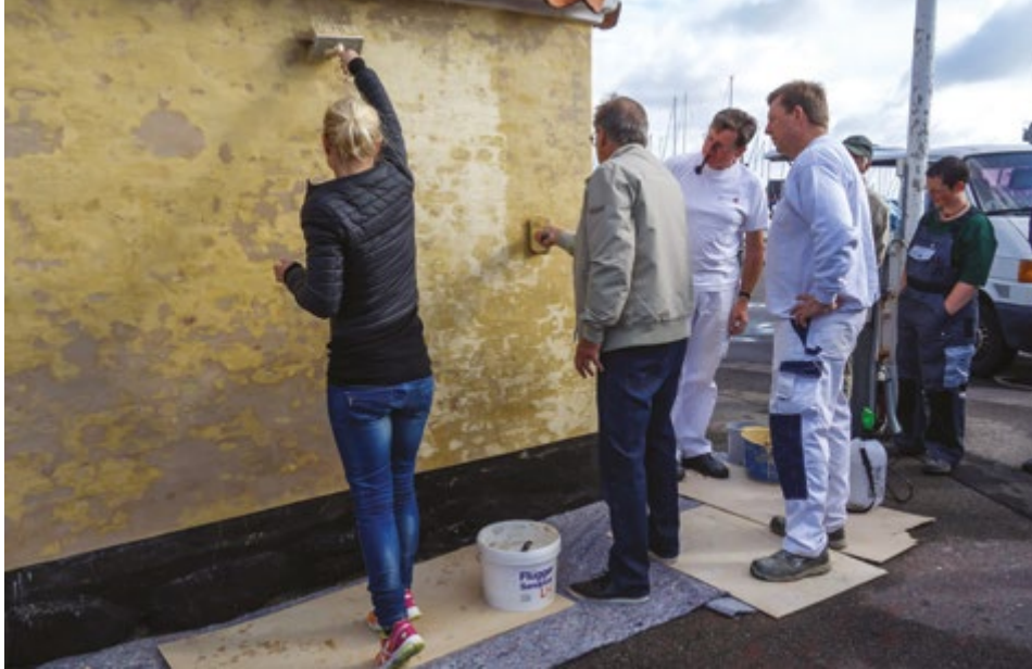
Dragør's house-owners applying lime-wash using traditional materials and techniques under the guidance of two craftsmen. Photo: Hanne Bendtsen, 2016
