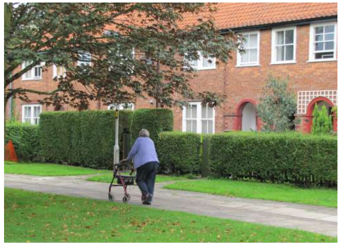
Above: New Earswick Village, built by Quaker industrialists as a model village near York, England . A garden city development from 1909, modernised to increase amenity for pedestrians by rationalising the road pattern.
