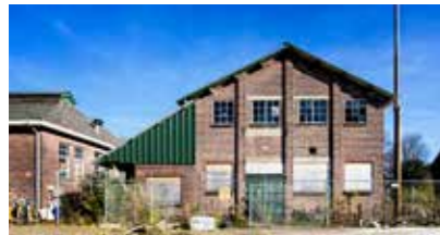
1909 Construction of power plant (Peel Power Plant)
