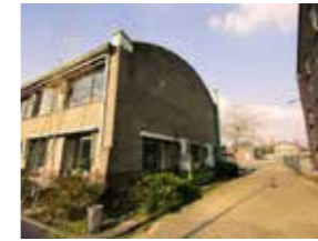
1950 Construction of blower room (Building 7)
