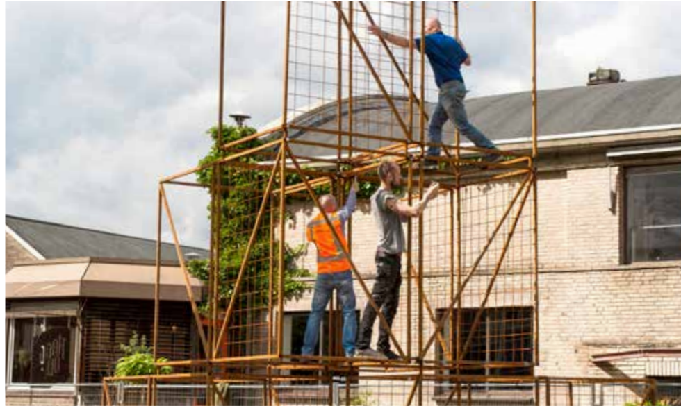
Temporary installation for Dutch Design Week
