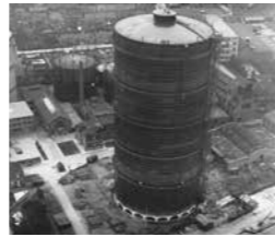
1941 Large gasometer is bombed
