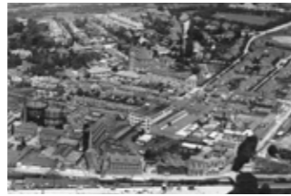
1925 Construction of garage (Building 17)
