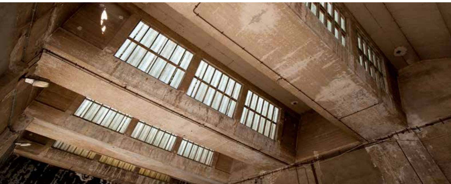
Interiors of buildings before renovation
