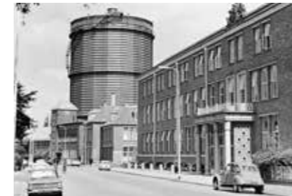
1946 Construction of Building 1 (offices)
