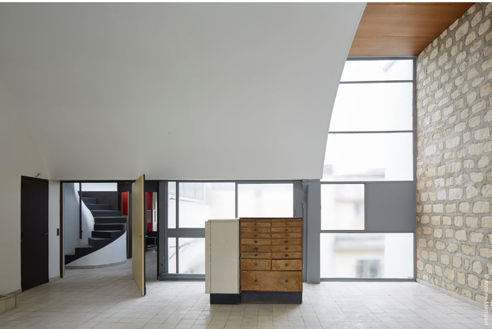
“Le Corbusier’s painting studio - interior vault insulated from the outside.” Le Corbusier Fondation.
