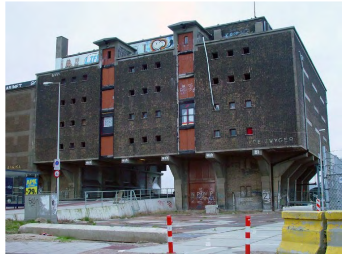
The Jan Schaefer Bridge was built through Pakhuis de Zwijger
