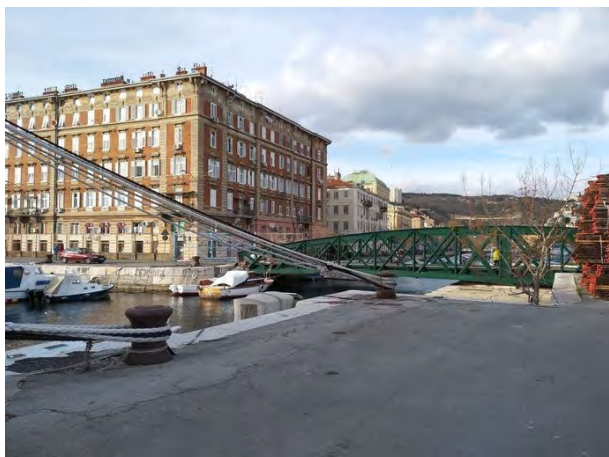
Figure 8: Movable Railway Bridge over Dead Channel
