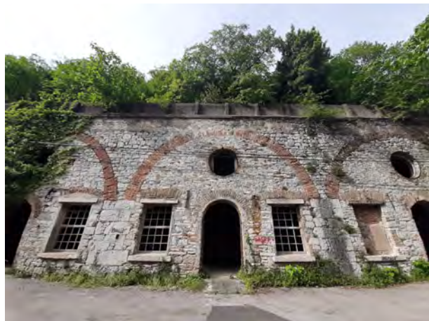
Figure 18: Aqueduct of Hartera Paper Mill
