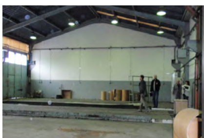
Figure 28: Dvorana kulture - Hall before renovation 2009. Source: Dvorana Kulture
