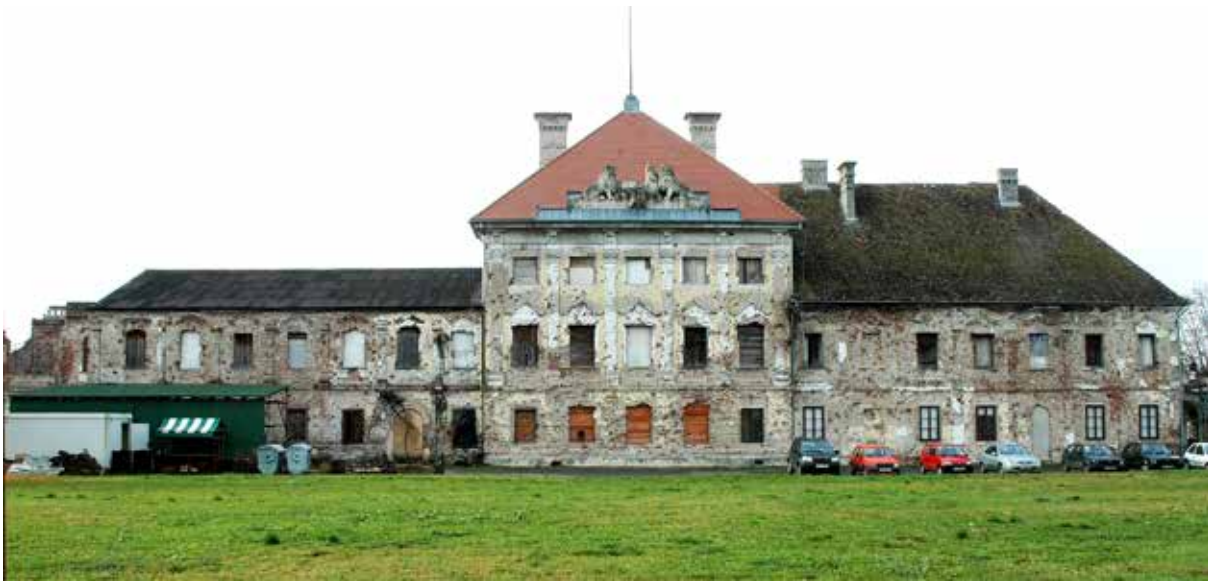
Eltz Manor, one of Meder's projects, at the beginning of the restoration. The castle was heavily damaged during the Battle of Vukovar in 1991 (photo by Mario Braun)
