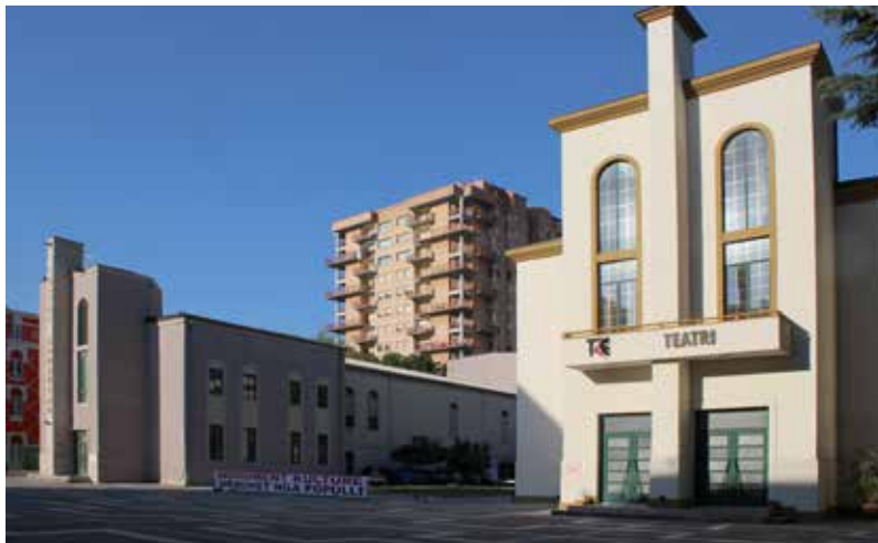
The National Theatre in Tirana, before its demolition
