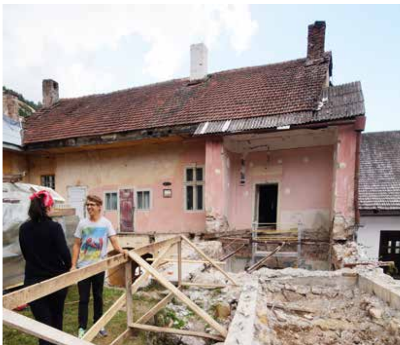
Casa Bocaniciu during restoration
