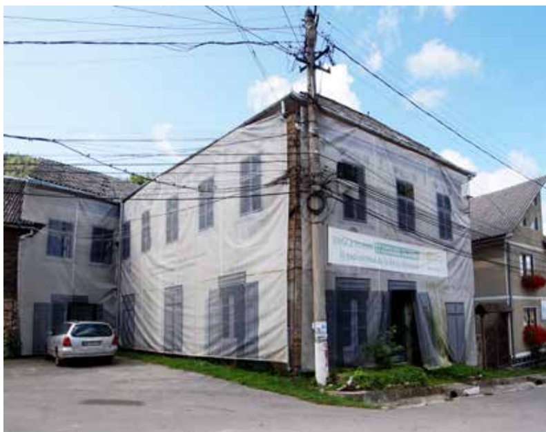
The town square of the village of Roșia Montană with houses covered in canvas
